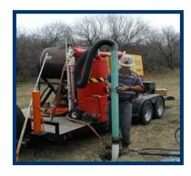
The Alpha Vacuum Excavation Process utilizes high pressure air to remove soil up to 12' deep in a safe and efficient manner around your pipelines. This system allows us to access finite locations on the pipeline without large excavation equipment and, in some cases, without the need for a one-call.
